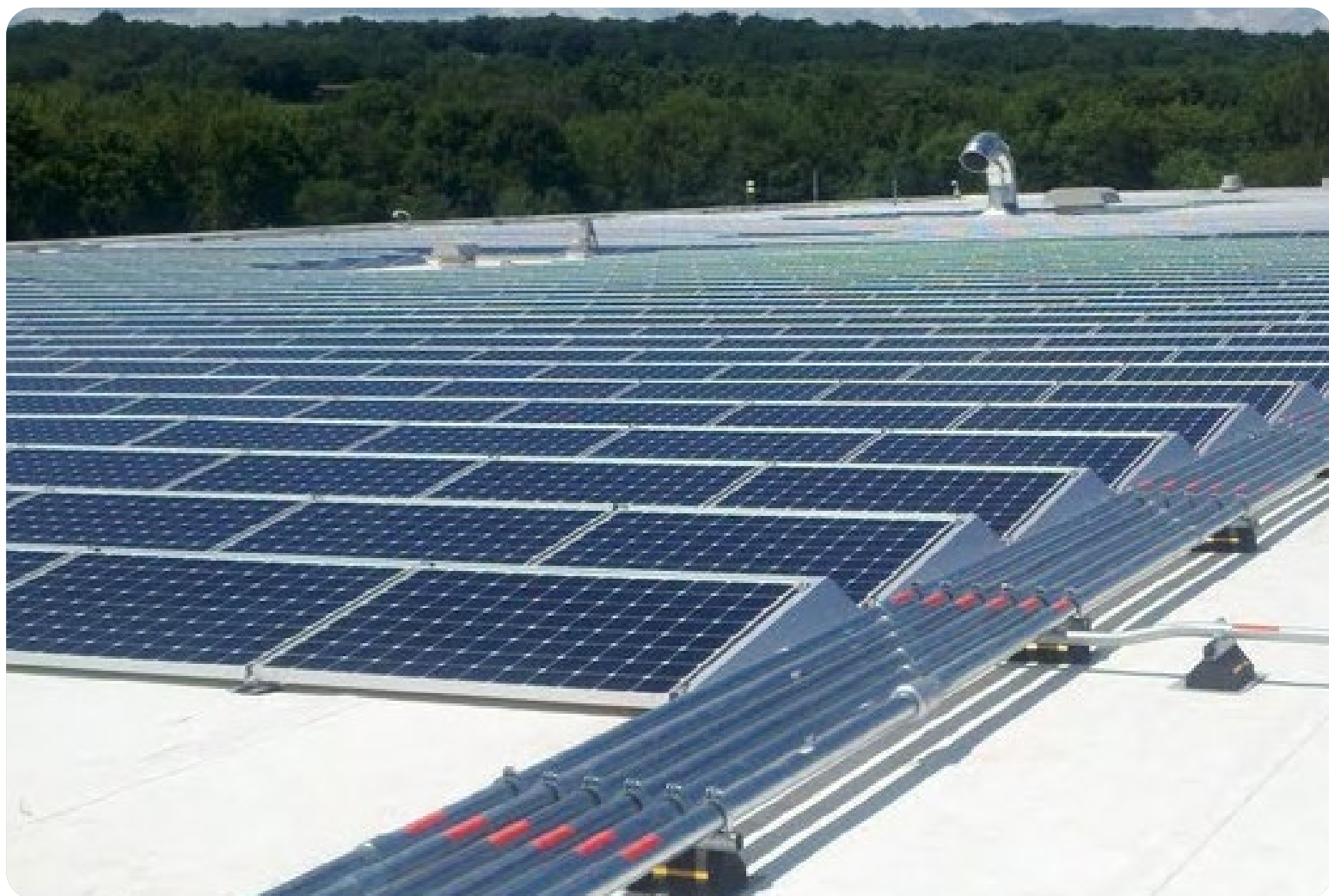
Skillman, New Jersey, Kenvue Administrative Offices
